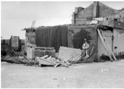
Fake Damage At De Havilland
